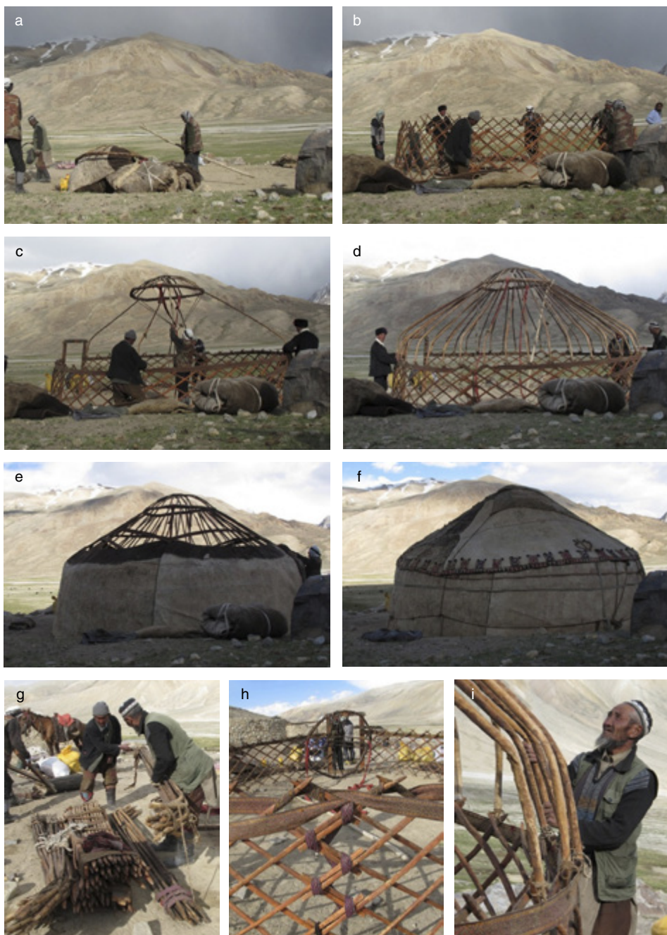
Fig. 1. Raising of a Kyrgyz yurt. a. Unloading. b. Setup of keper. c-d. Fitting of wuuk and tündük. e. Fitting of felt-covers. f. Complete. g. The entire wooden construction collapsed. h. Straps. i. Headman Muhammed Ayoub fitting a wuuk-pole.
